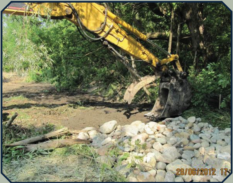
Ditch fill being smoothed at Valley Woods Wetland.
